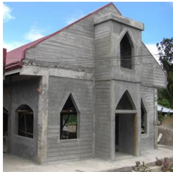
Church under construction.
