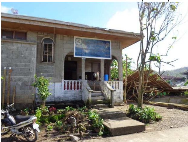
Church in a house. The Front is still standing.
